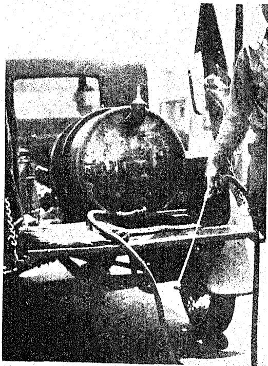
Figure 68. Pressure oil barrel on a light truck, used in oiling underground street vaults and street inlets
